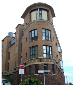
Synthetic Building of the School of Chemistry at the University of Bristol
